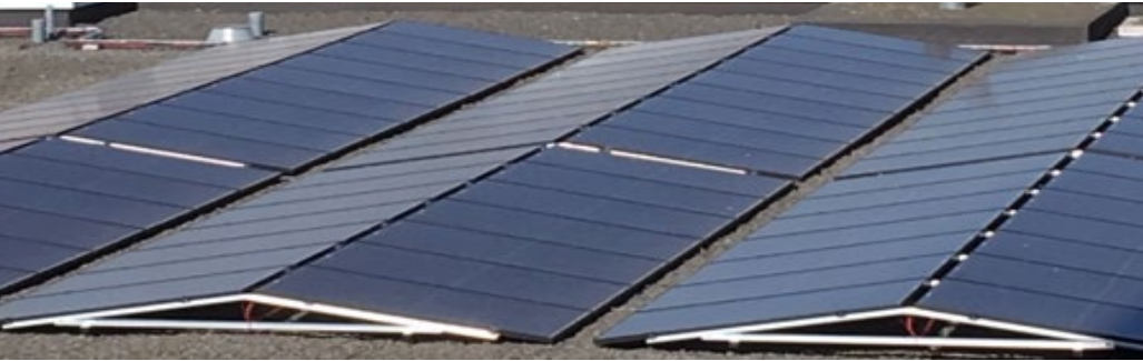
Figure 5 - Example of solar PV installation on a flat roof (orientation towards east/west)
